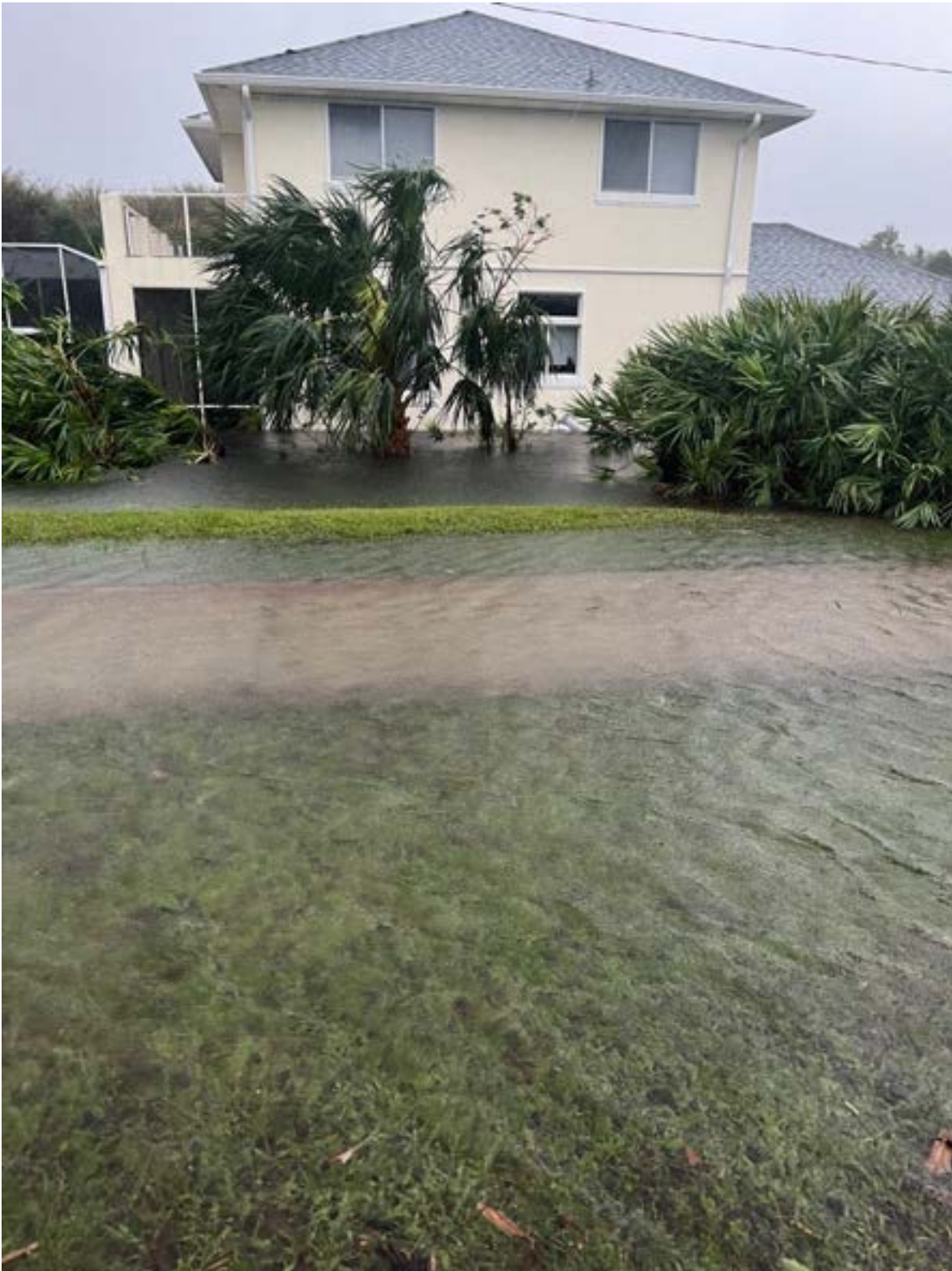
Figure 11. Hurricane Ian Flooding at Southwest Corner of Coastal Oaks Circle and S Atlantic Avenue
