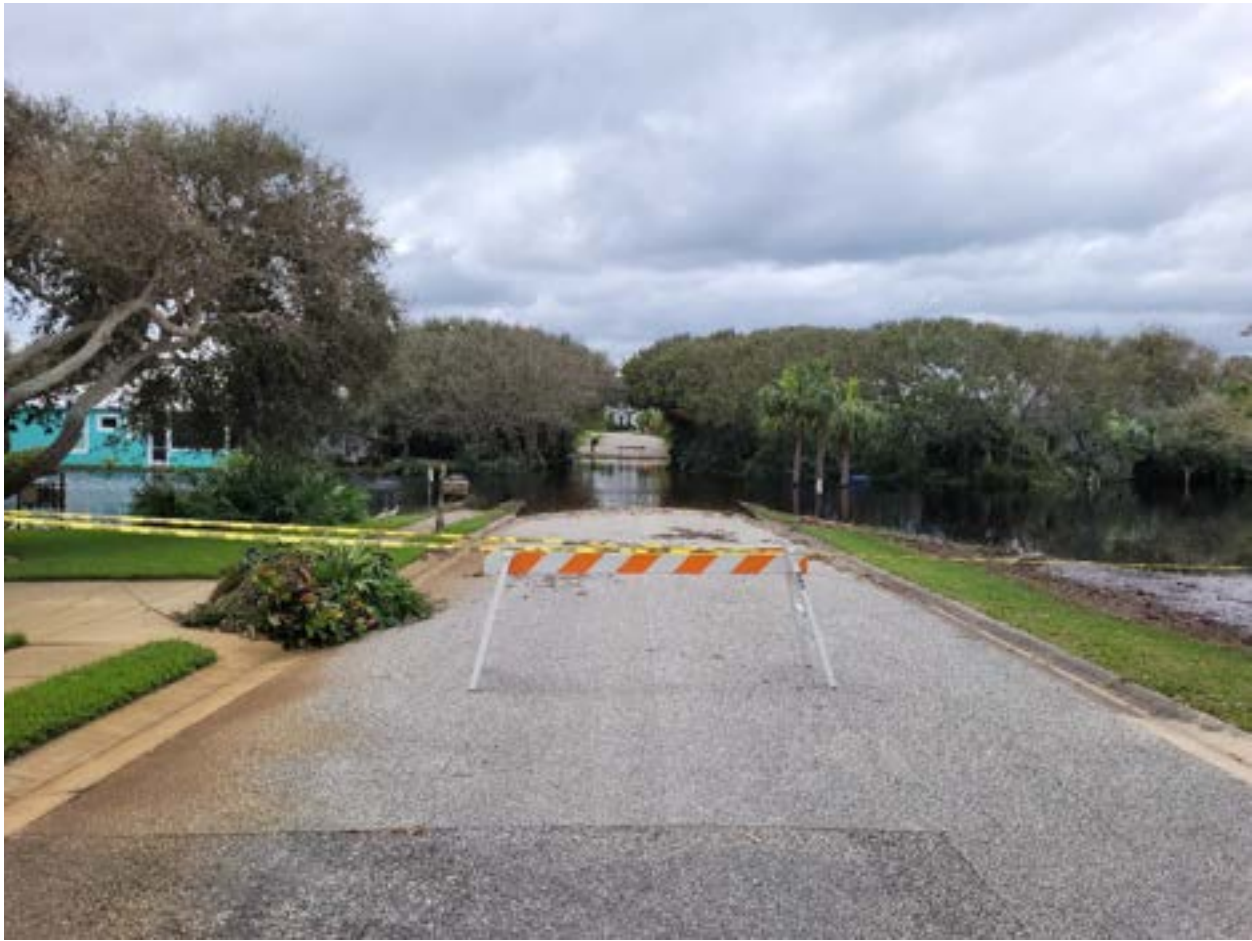
Figure 15. Hurricane Ian Flooding on Inlet Point Boulevard Facing West
