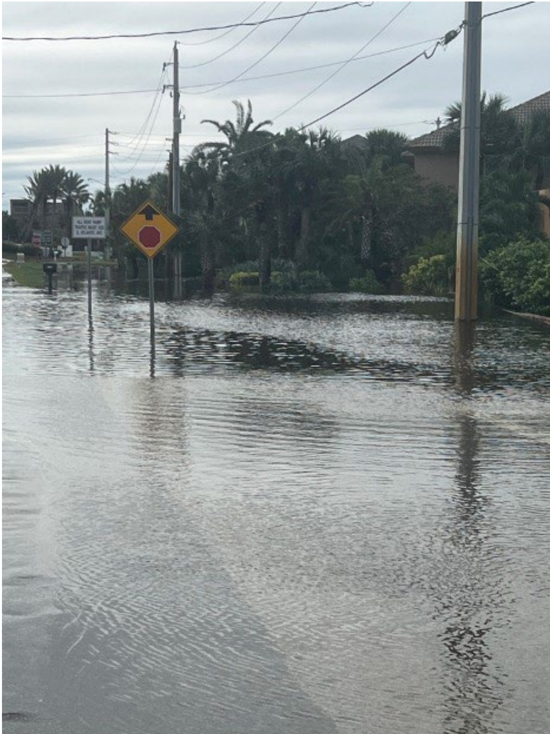
Figure 12. Hurricane Ian Flooding on S Atlantic Avenue at Inlet Point Boulevard
